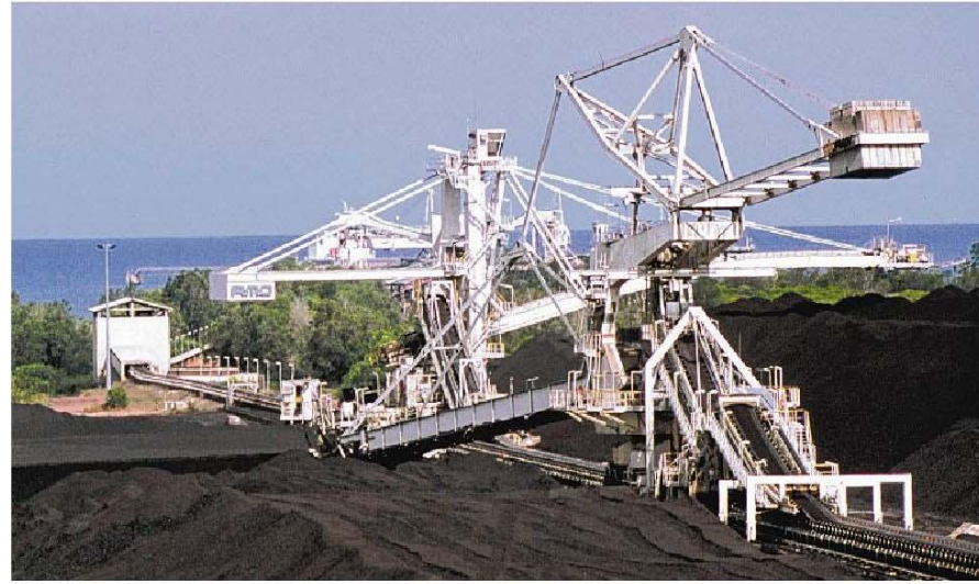
Coal mine in East Kalimantan, Indonesia. While there has been much debate about green finance, transition finance is more relevant to South-east Asia given that many economies have yet to fully adopt clean energy and wean themselves off fossil fuels. PHOTO: BLOOMBERG
