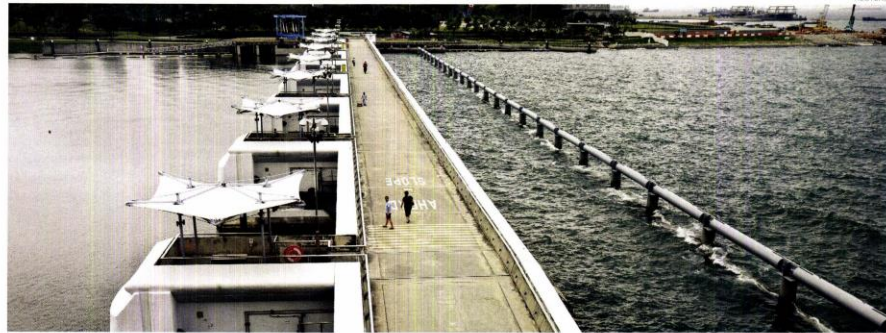
The Marina Barrage pumps water out of Marina Reservoir into the sea when it rains heavily. PUB plans to build a second pump house at the opposite end of the barrage.
