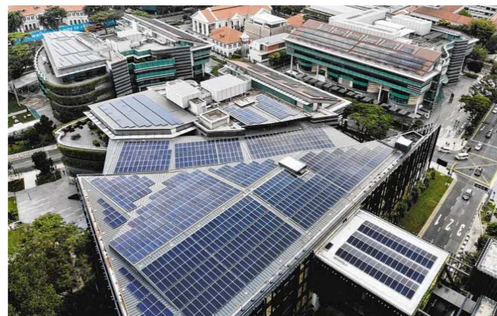
SMU has the largest on-site solar farm in Singapore's city centre. PHOTO: SINGAPORE MANAGEMENT UNIVERSITY
