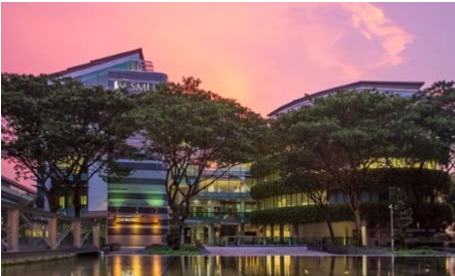
Li Ka Shing Library at Singapore Management University. Photograph: Hong Huazheng
