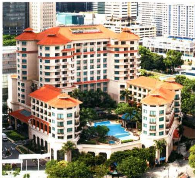
After refurbishment to make it more environment-friendly, Swissôtel Merchant Court can expect energy savings of more than 2.28 million kWh per year and a reduction in water usage by some 6,460 cu m
