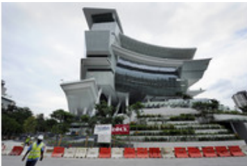
The Star Performing Arts Centre nears completion in Singapore. Photographer: Munshi Ahmed/Bloomberg
