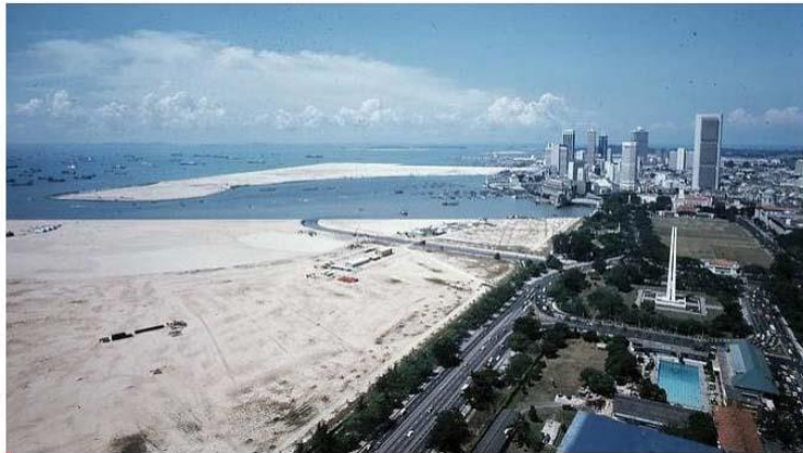
Reclamation work at Marina Bay in 1977. (Photo: Urban Redevelopment Authority)
