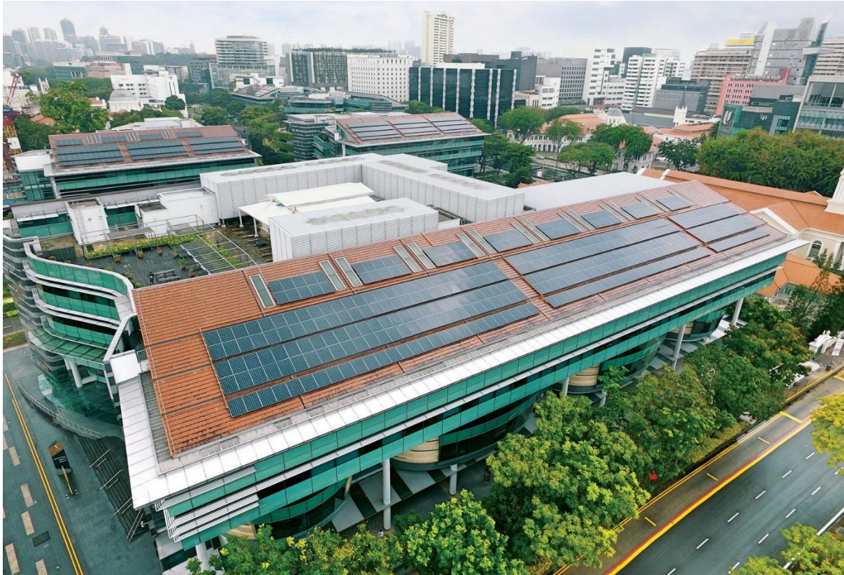
Solar panels atop one of SMU's buildings. PHOTO: SINGAPORE MANAGEMENT UNIVERSITY
