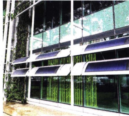
Energy-saving features such as solar chimneys that suck warm air (left) and shading devices (right). TNP PHOTOS: JONATHAN CHOO
