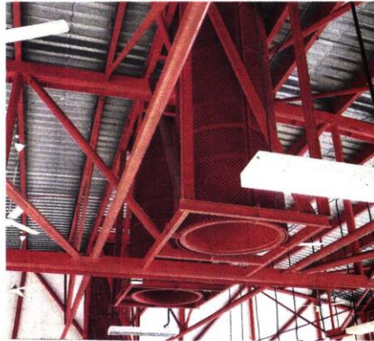
Energy-saving features such as solar chimneys that suck warm air (left) and shading devices (right). TNP PHOTOS: JONATHAN CHOO
